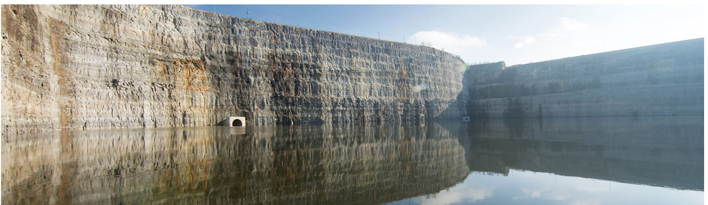
TARP Reservoir, Credit: MWRD
