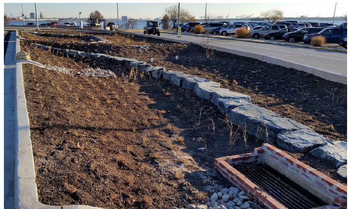
Vegetated stormwater basin in parking lot after planting. Credit: Blue Water Baltimore
