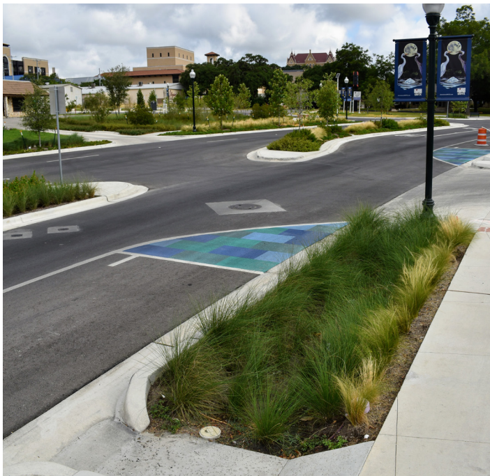
CM Allen Parkway after completion. Credit: City of San Marcos
