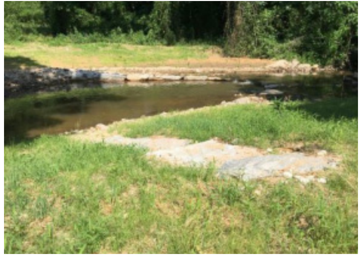
Mill Creek erosion control. Credit: EPA
